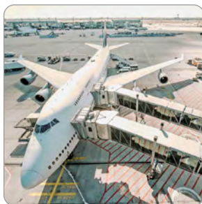
旅客登机桥 Passenger boarding bridges
