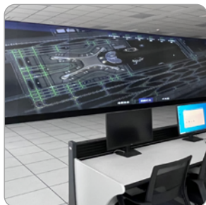
ALCMS-C 助航灯光监控系统 ALCMS-C Airport Lighting Control and Monitoring System
